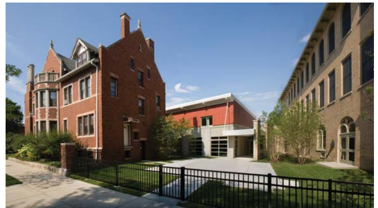
Holabird & Root planned, programmed, and rehabilitated a 30,000-sq.-ft. former Catholic school and church (above) to convert it into the Concordia Avondale Campus Community Center (top) with an early childhood education program as well as multipurpose spaces for school-aged children, teens, and seniors. Photography by James Steinkamp.
