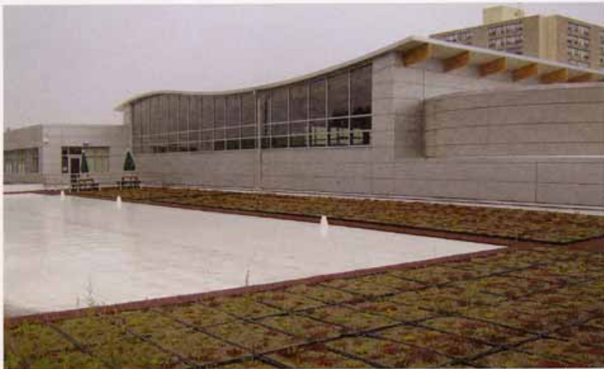
Among the building's green features is the living roof, 10,000 square feet of vegetated space with white membrane covering the remainder.
