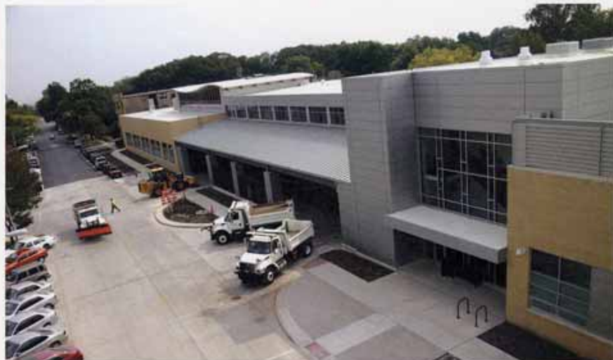
The new 155,000-square-foot Public Works facility for the Village of Oak Park will likely become a model for future projects in the region.
